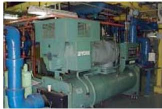
water away from some industrial process which has heated the water. The chilled water can then be used to cool and dehumidify air in mid- to large-size commercial, industrial, and institutional facilities. Most chillers are designed for indoor operation, but a few are weather-resistant.
